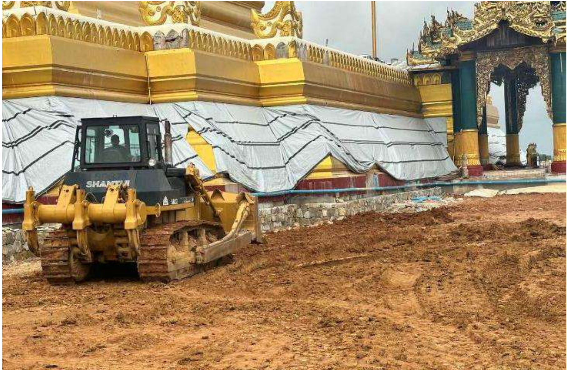
Uppathasanti pagoda in Nay Pyi Taw conservation work
