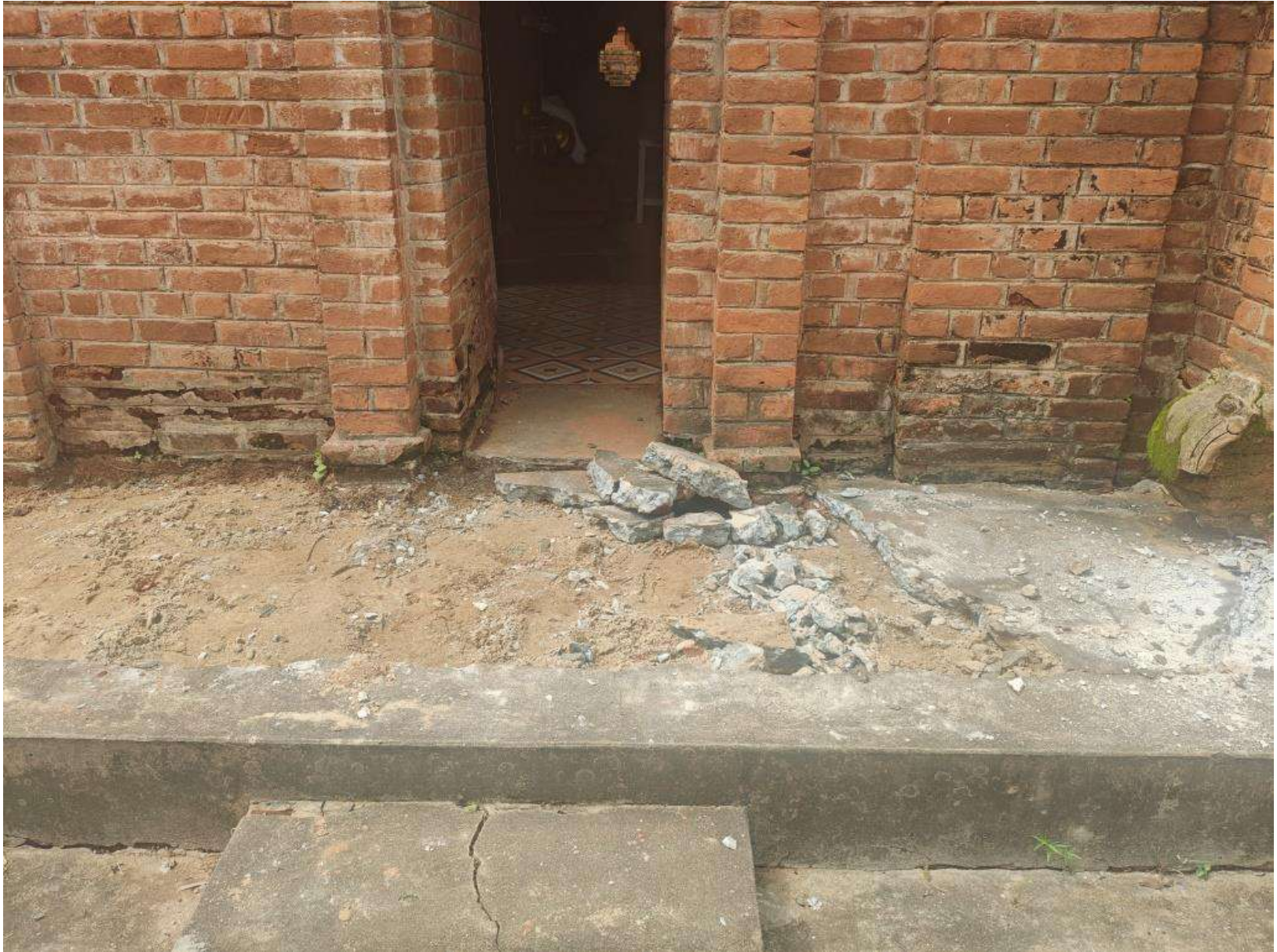
Sima in Nay Pyi Taw-Bagan Pagoda Complex before restoration work
