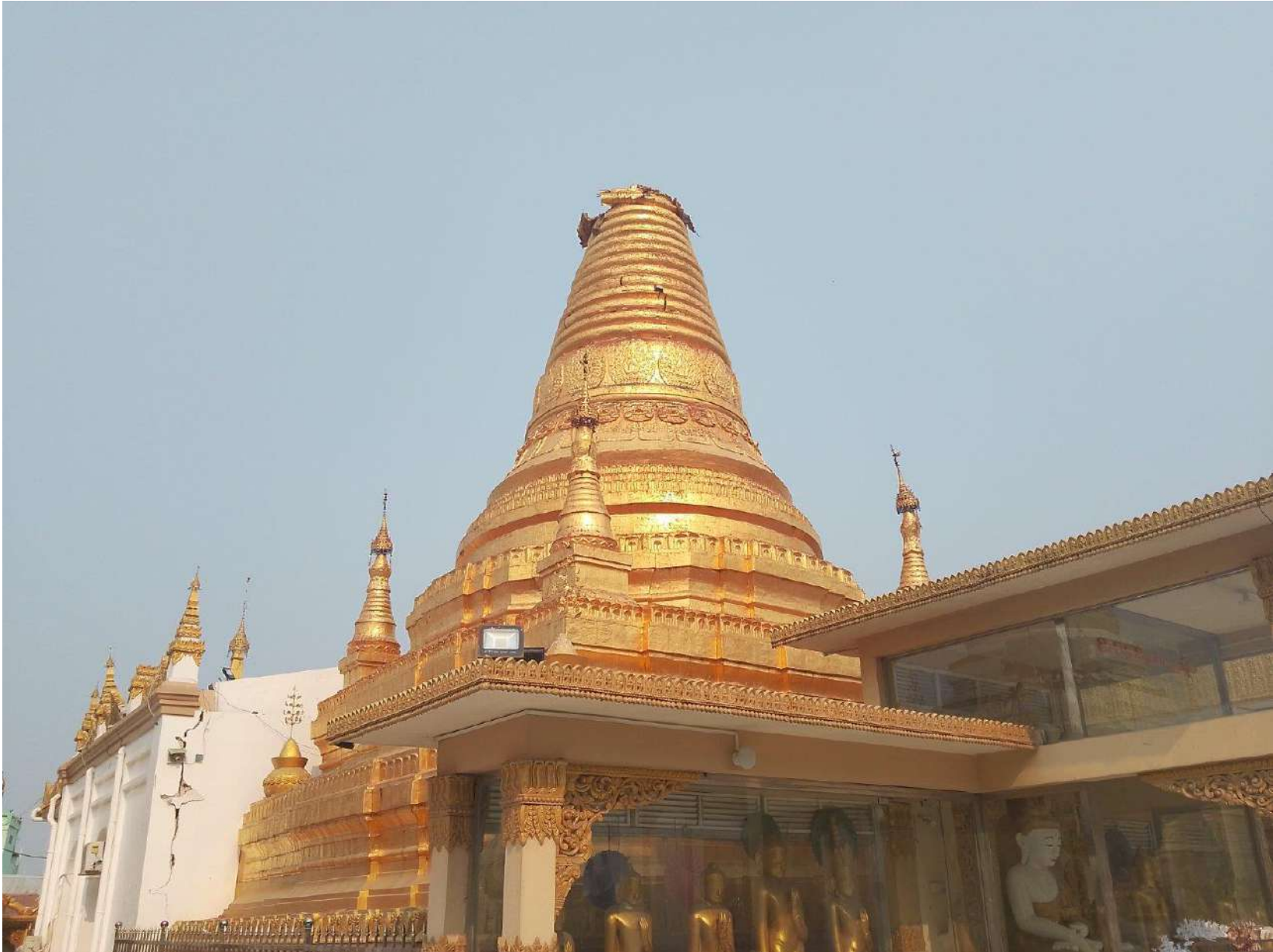
Sel Taw Na Shwe Moat Htaw Stupa in Kyaukse before restoration work
