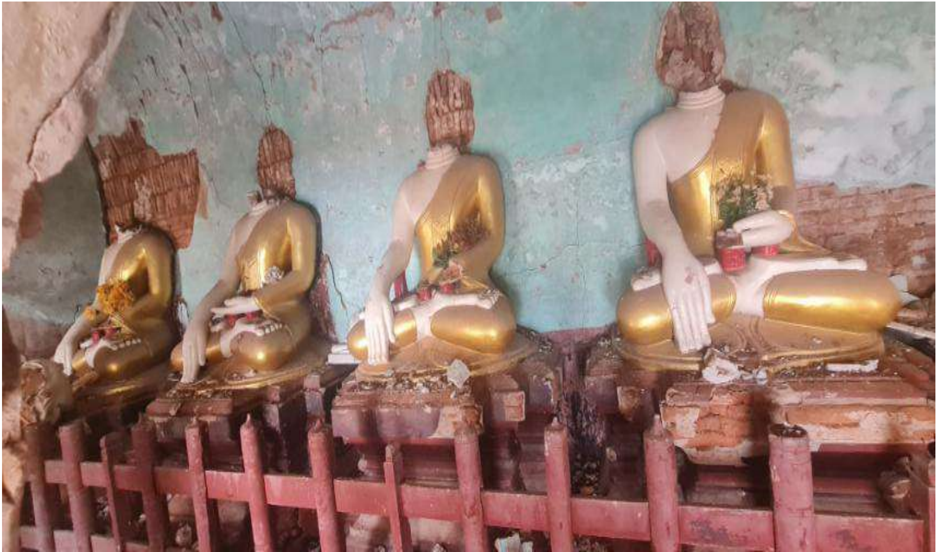
Five Pagodas (Ngar Su Phayar) in Makkhara before restoration work
