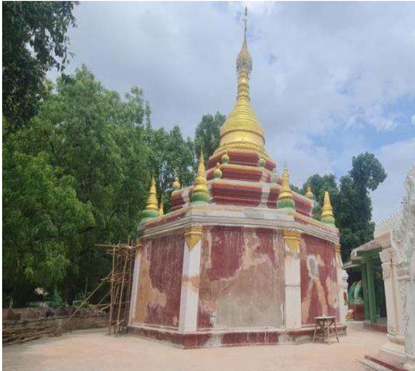
Shin Pin Ku Hla in Paleik restoration work
