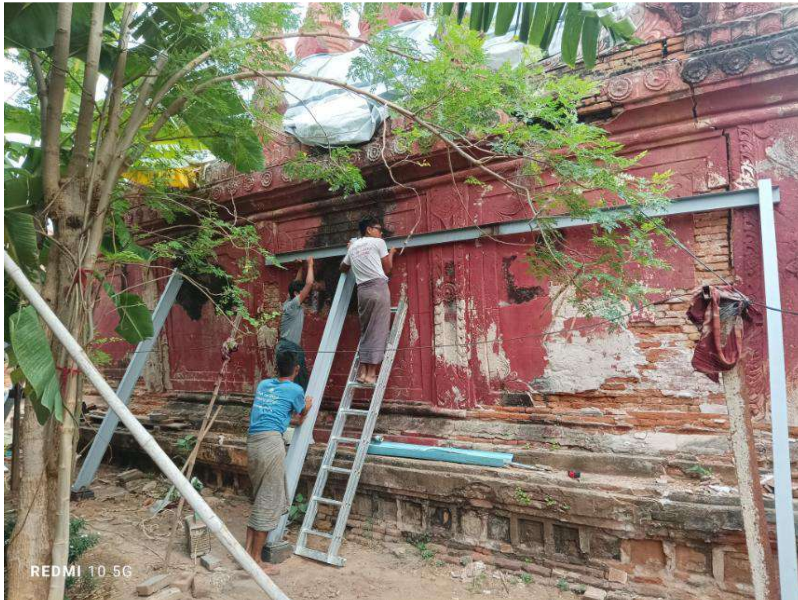
Five Pagodas (Ngar Su Phayar) in Makkhara before restoration work
