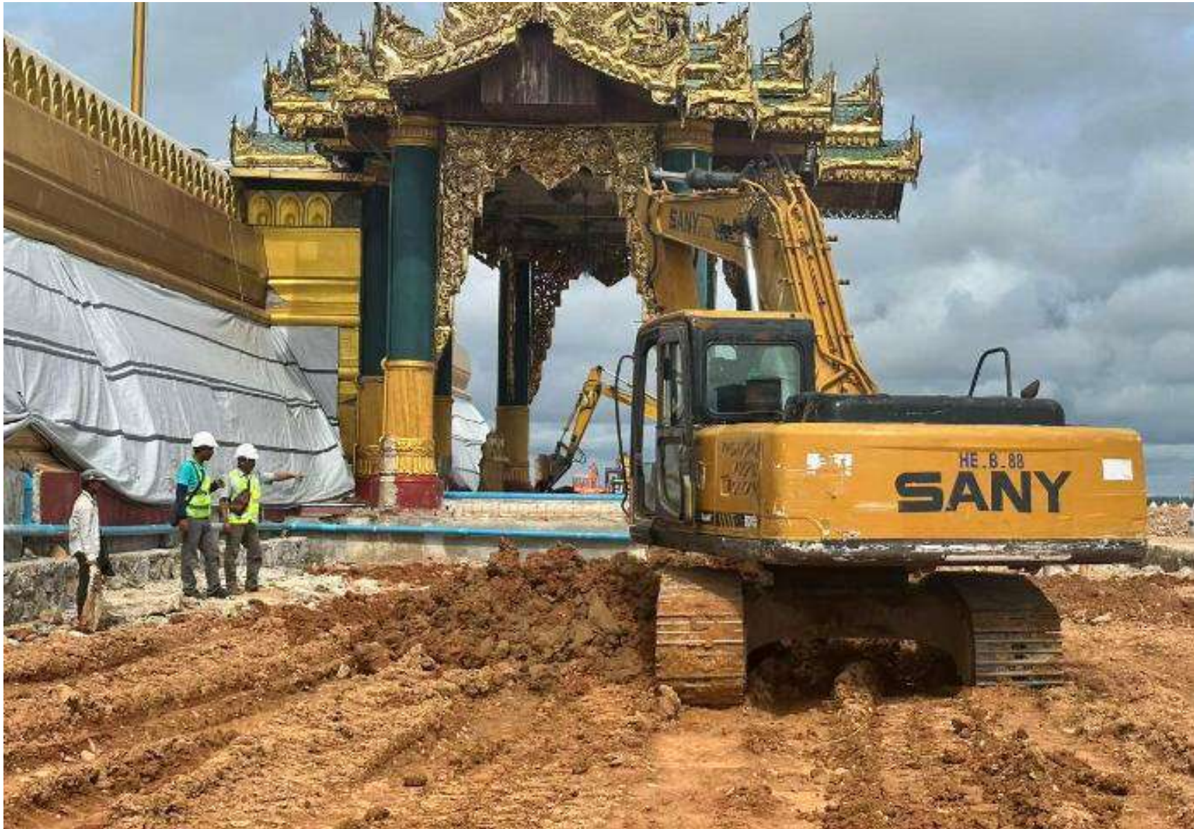
Uppathasanti pagoda in Nay Pyi Taw conservation work
