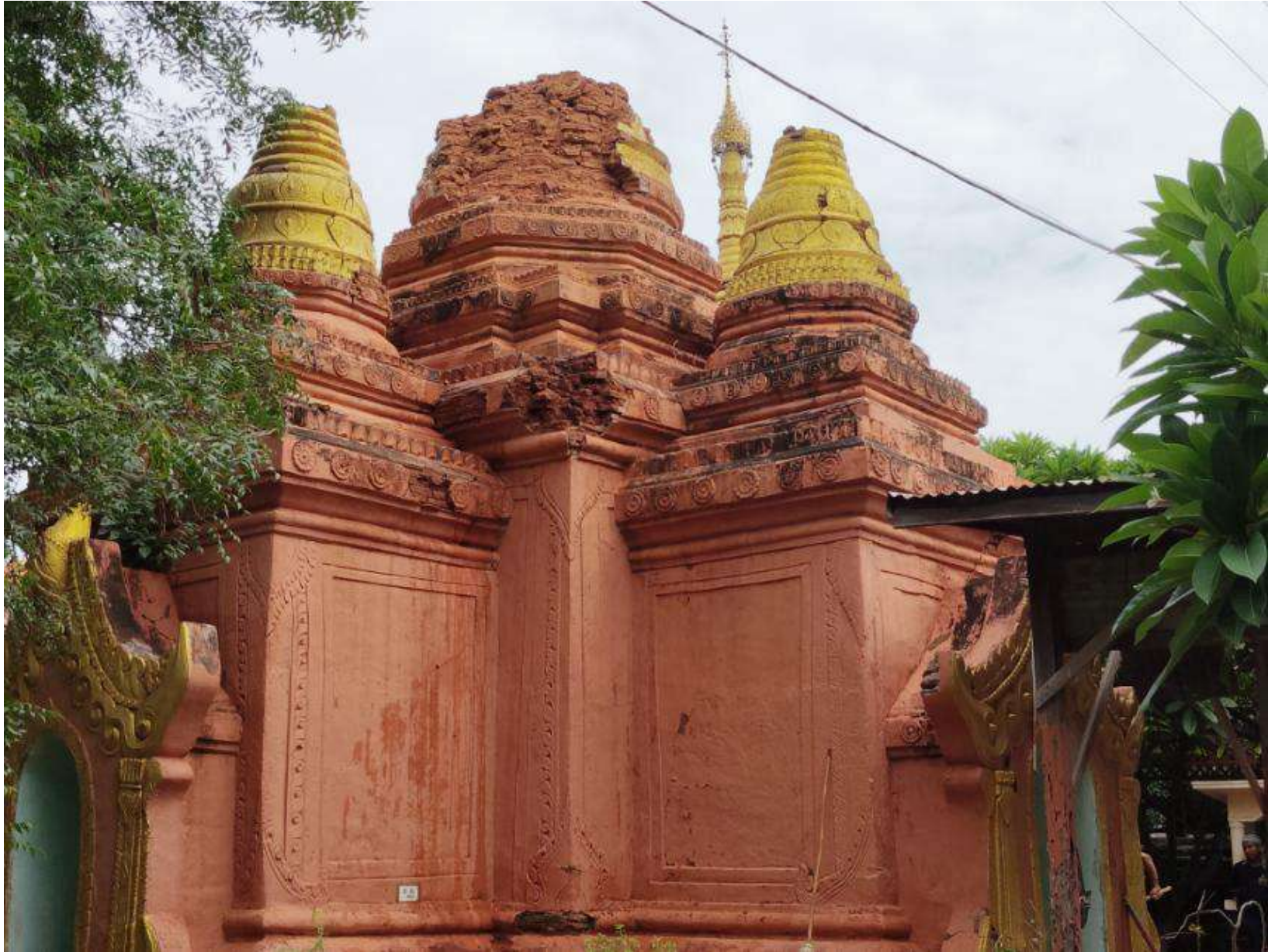
Sayh Stupa in Makkhara before restoration work
