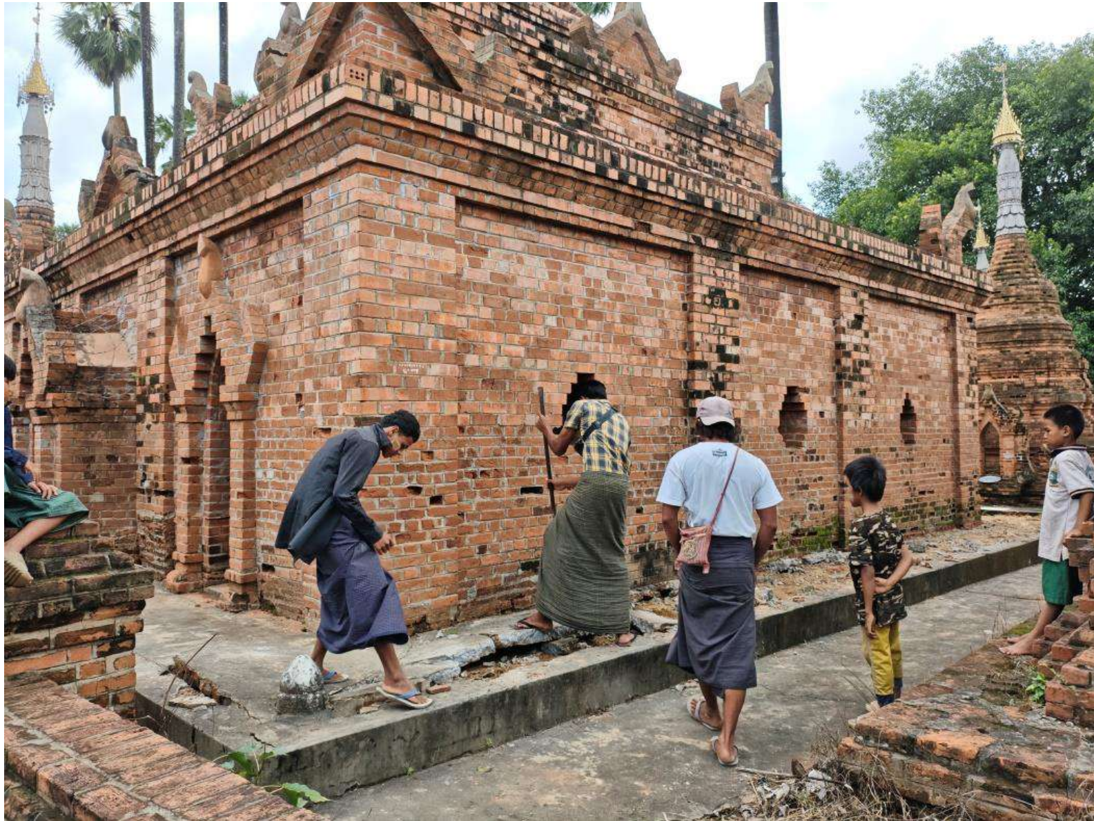
Sima in Nay Pyi Taw-Bagan Pagoda Complex during restoration work
